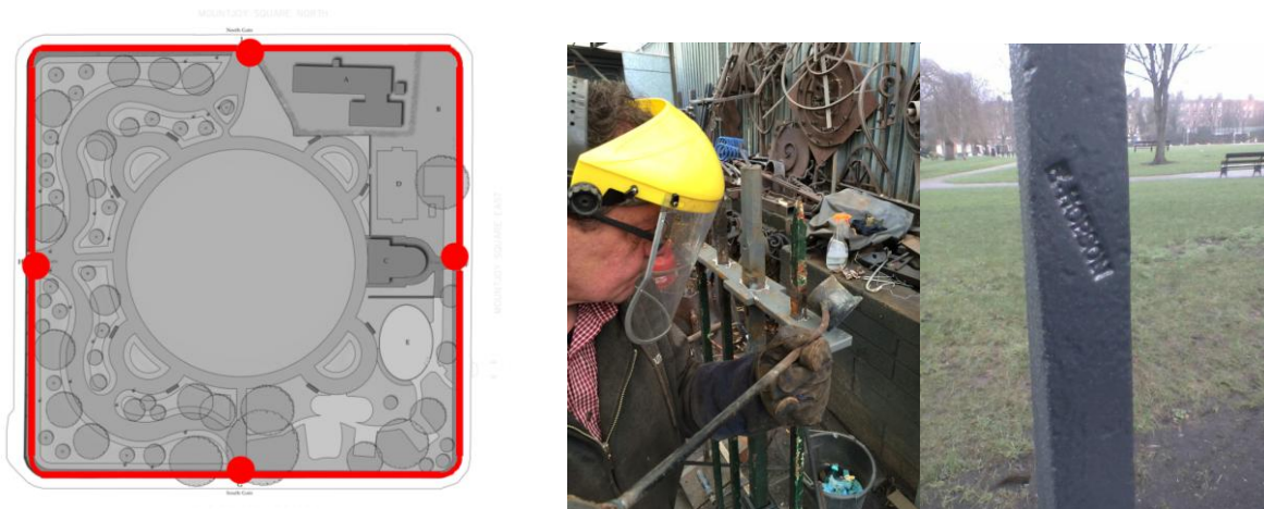
Figure 9: Wrought iron railings refurbishment
