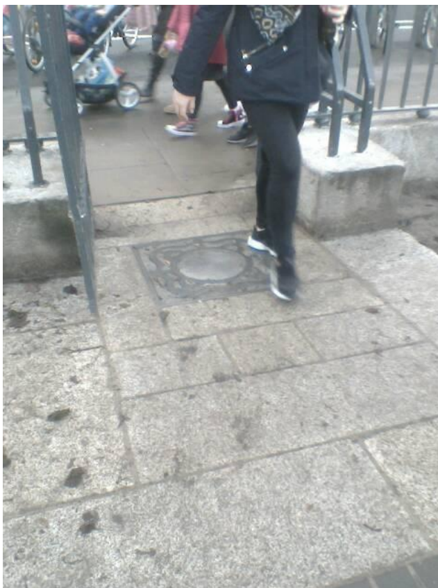
Figure 13. Paving upgrading at the west gate which will also be installed at other gates around the park
